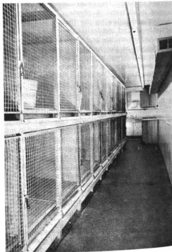
FIGURE 14.3B. (Right) Interior view showing full length of animal trailer used in the Fission Product Field Release Tests at the National Reactor Testing Station. Beyond the dog cages at the far end is a furnace-air-conditioner, water heater and storage facilities. Normally cages for rats were mounted on the right wall. (The usual practice of not mixing species in animal care facilities was not employed because of the relatively short duration of the experiments.) (Courtesy of Wilson 1959.)
